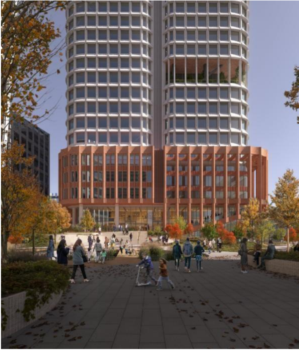
Figure A: Indicative view of Regent's Place Plaza
