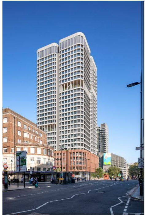
Figure B: View from Tottenham Court Road at Grafton Street of revised proposals
