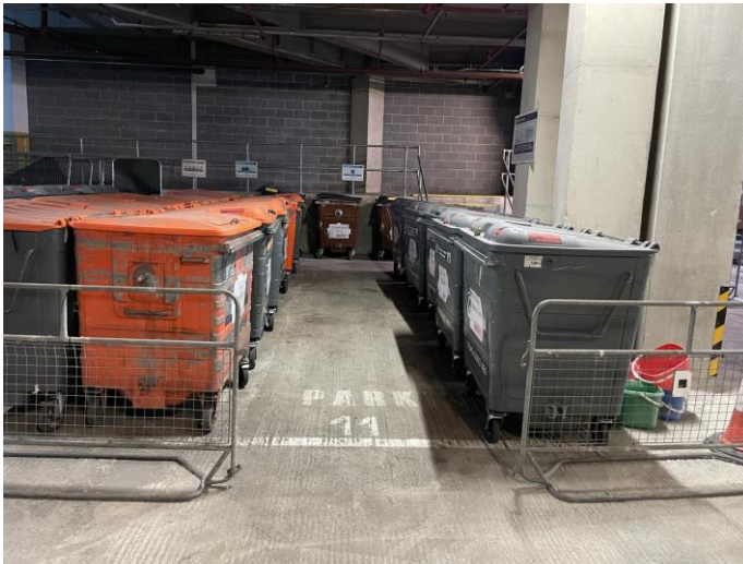
Figure 3-1 Typical Service Yard Waste Storage Area
