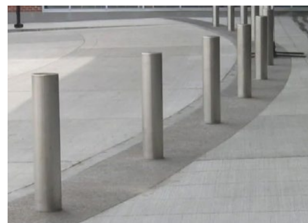
01 When there is the absence of a mound, the security line is supported by 900mm ht. bollards.
