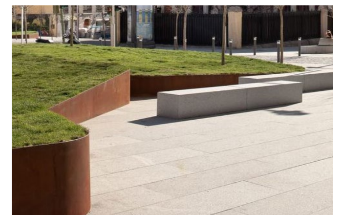
02 Throughout the design, large mounds shape the landscape, offering additional security support through their height and immovability. These planters will have an external planter wall height of min. 650mm.
