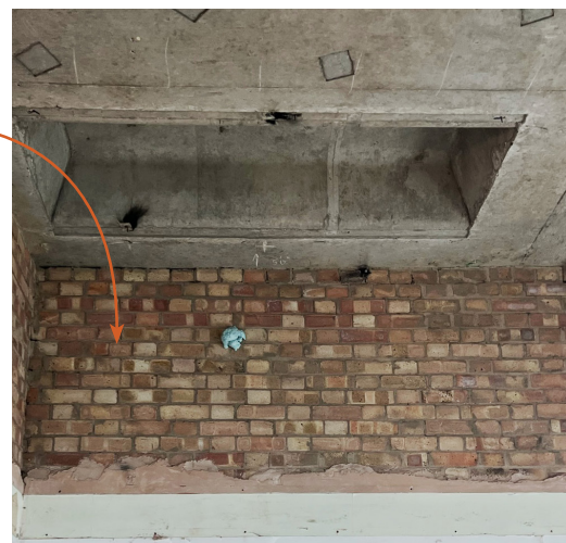
Figure 4.27 Brickwork used within existing cores at Euston Tower
