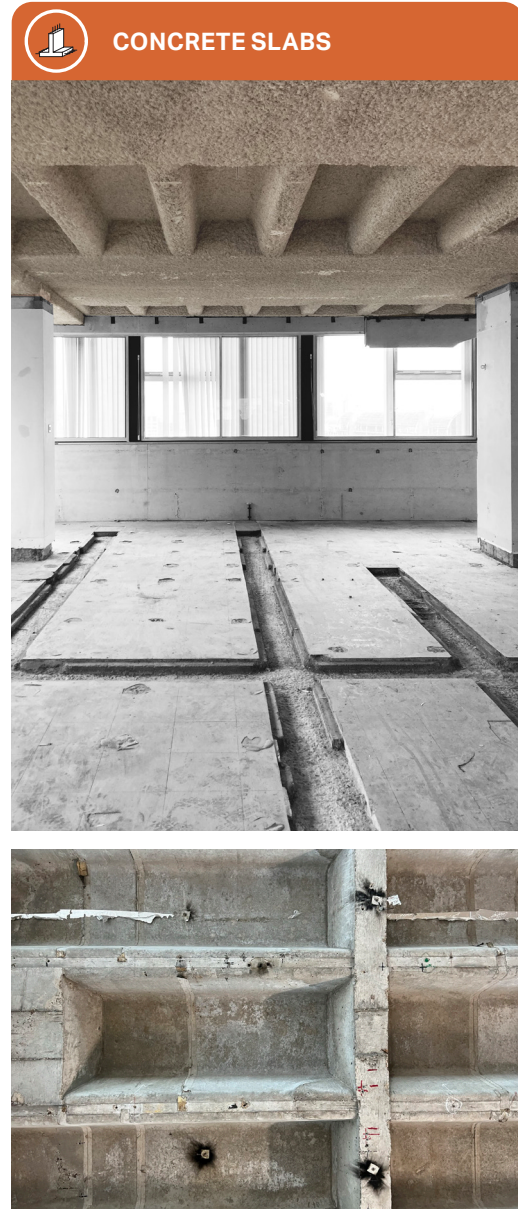
Figure 4.3 Ribbed concrete slabs at Euston Tower
