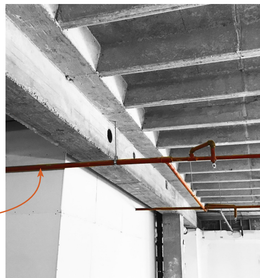
Figure 4.22 Levels 01 and 02 fire sprinkler pipes at Euston Tower
