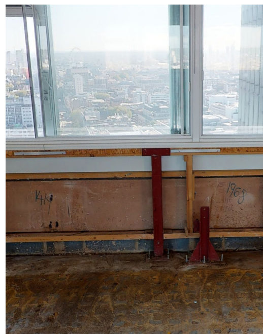
Figure 4.32 Timber in facade substructure at Euston Tower
