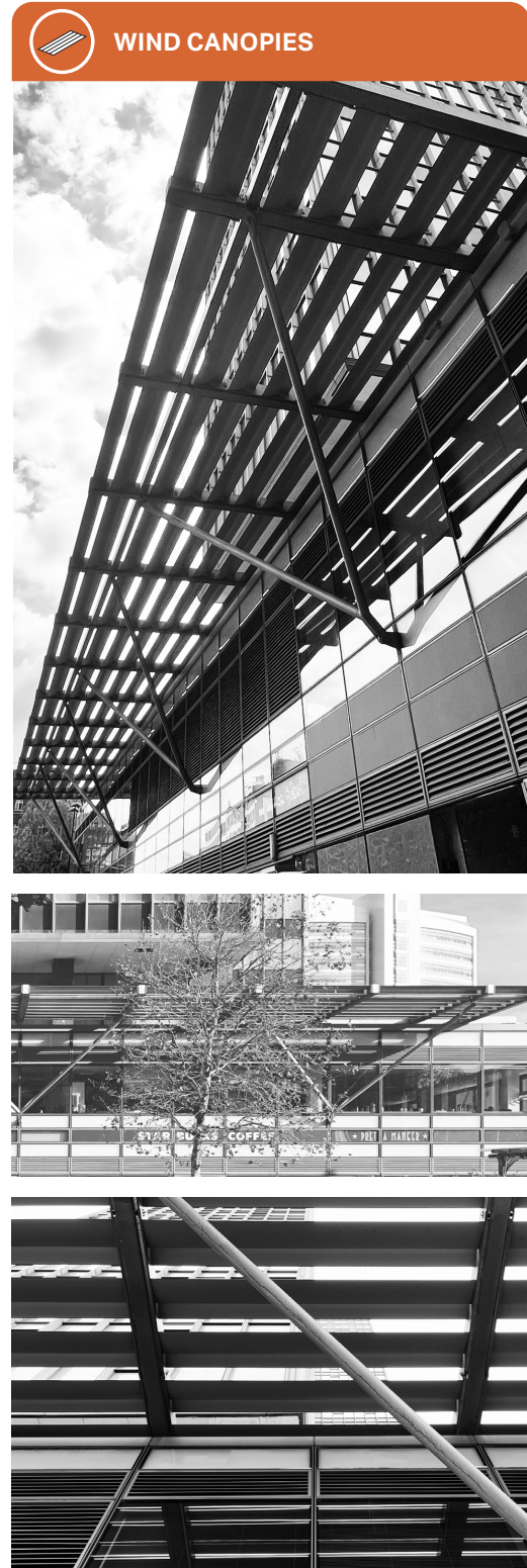
Figure 4.18 Existing podium wind canopy at Euston Tower
