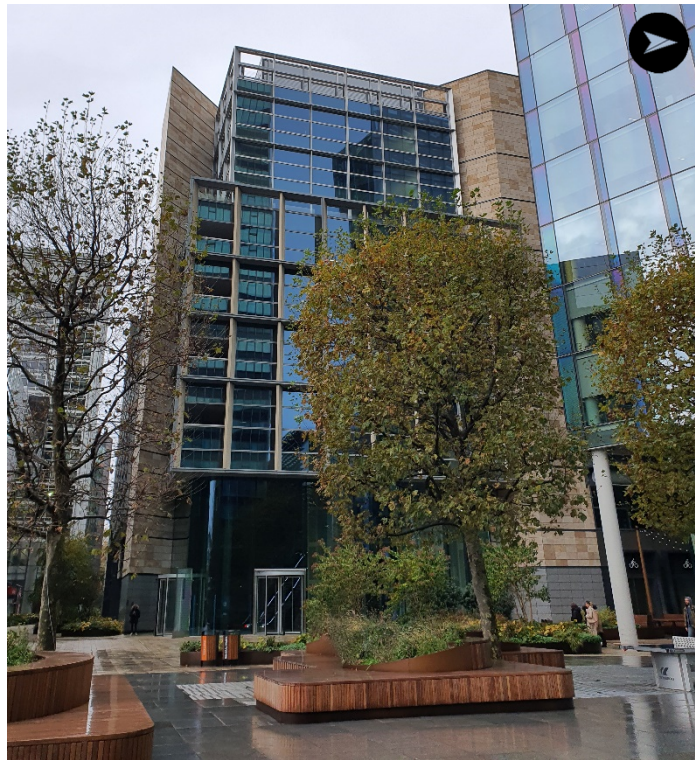
Figure 3: 1 Triton square looking west from Euston Tower (image taken 10/11/2023, Arup)
