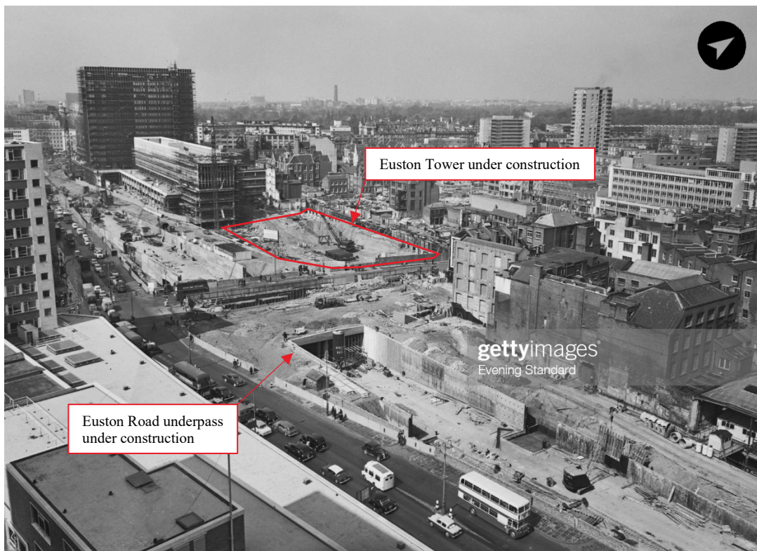
Figure 7 - Euston Road underpass under construction (Evening Standard, 1965)
