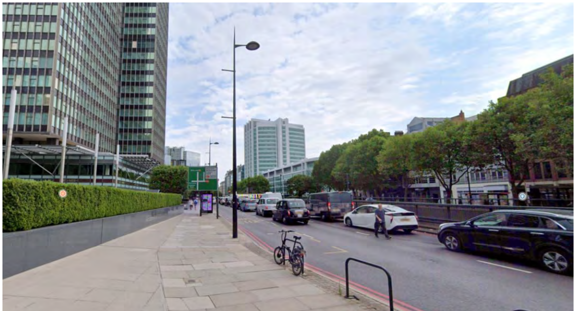
Figure 8-8: Euston Road off-slip Bus Stop
