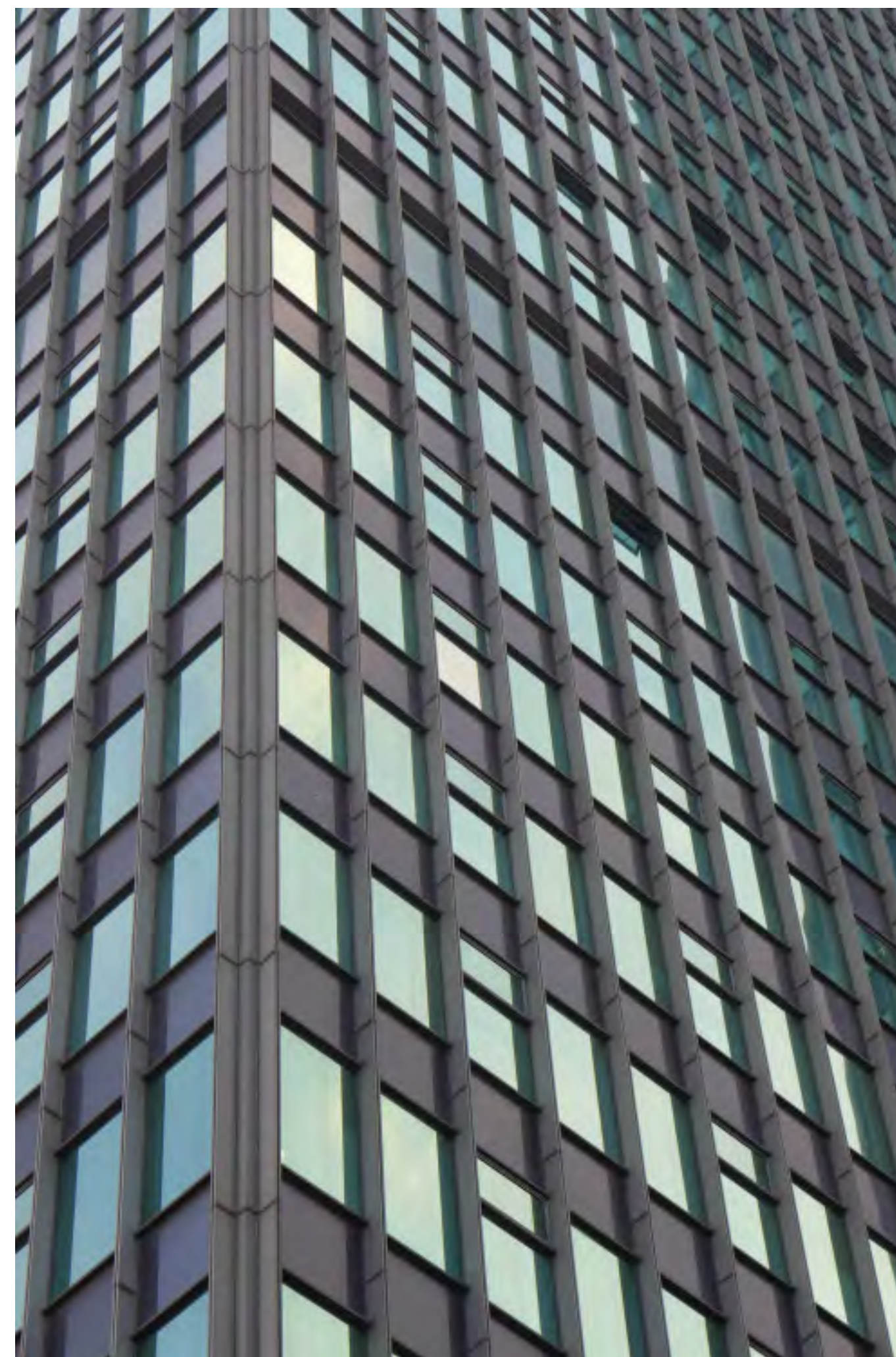
Figure 9: View of the Euston Tower's curtain walled façade
