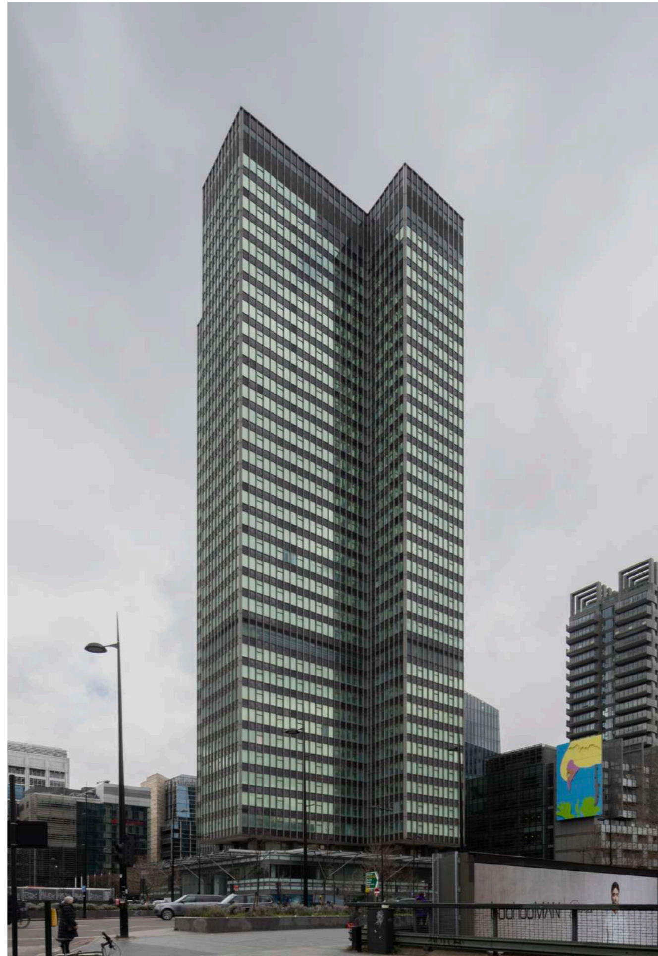
View from Euston Road - looking west
