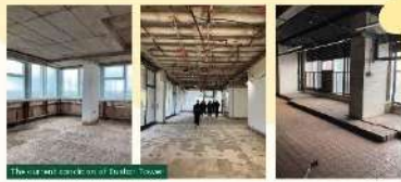
The old section of Fusion Tower
