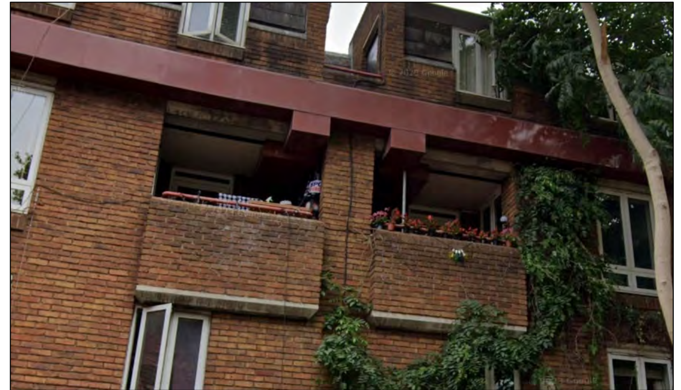
Figure 11.10 Tolmer's Square – Street View of Residential Recessed Balconies
