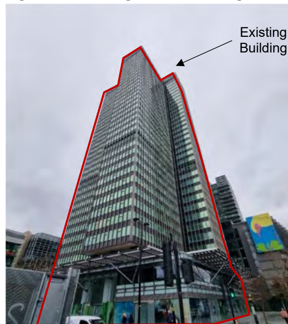
Euston Tower, photo taken from the junction of Hamstead Road and Euston Road.
