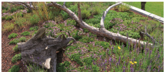
Section and precedent of biodiverse roofs illustrating a range of substrate and habitat features.
