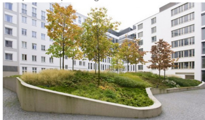
Reference: Delfland Water Authority, The Netherlands
