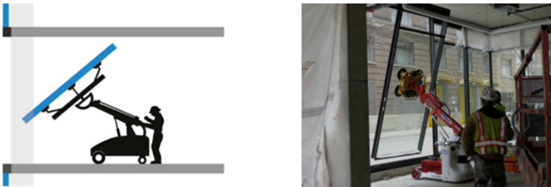
Figure 9.23 Installation of window-wall facade
