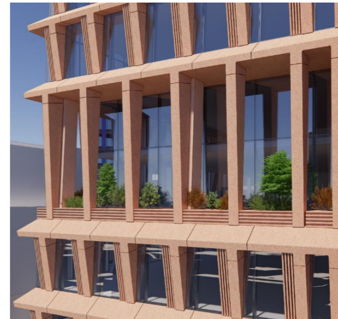
Figure 8: Example of amenity space glazing adjacent to a terrace area showing shading provided by the projecting storey above, planting and the structure.
