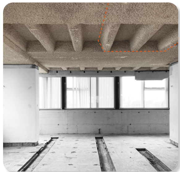
Figure 3.13 Reference photo for example slab location
