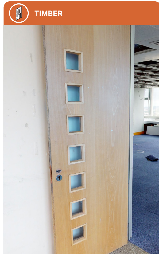
Figure 4.33 Existing timber doors at Euston Tower
