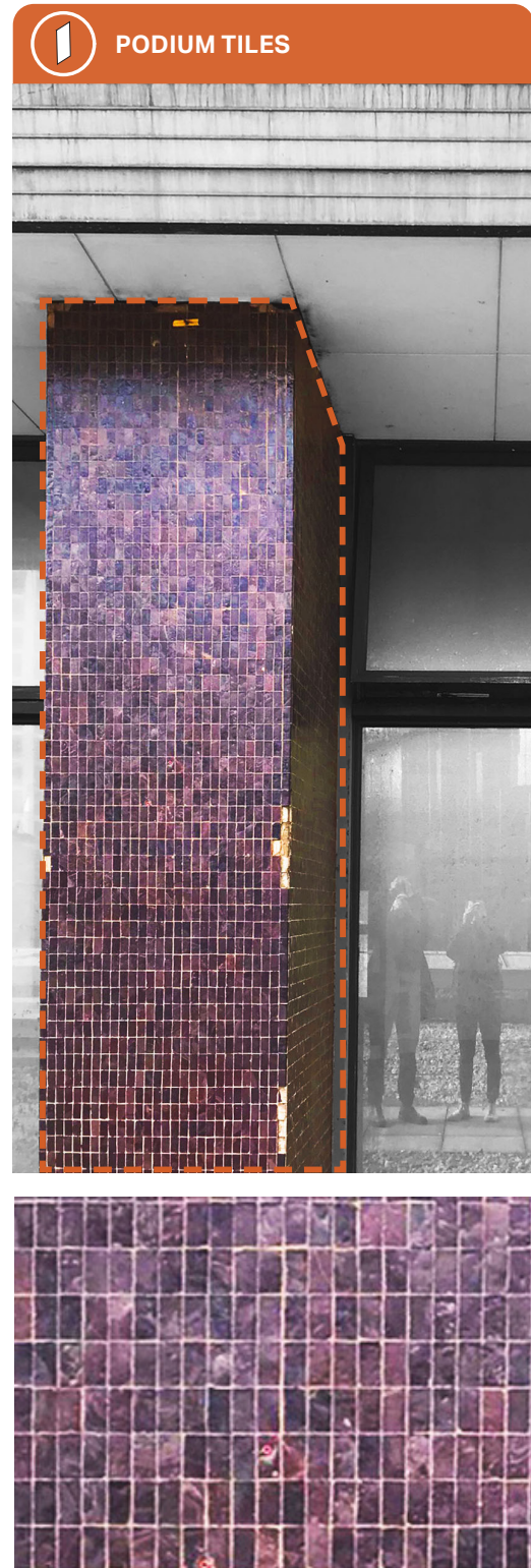
Figure 4.15 Existing red tiles on external podium at Euston Tower
