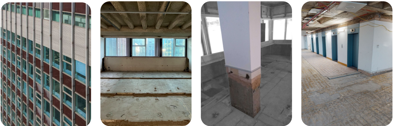
Figure 3.1 Images from existing building showing its current condition
