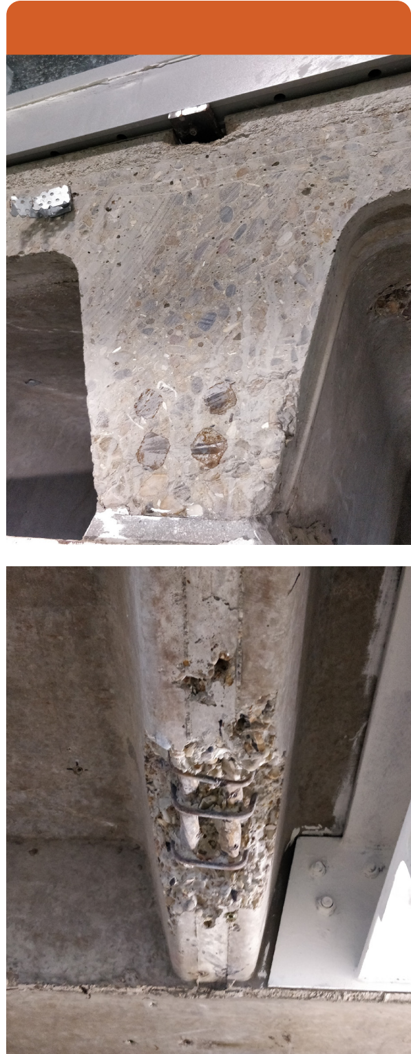
Figure 3.8 Images of existing ribbed slabs
