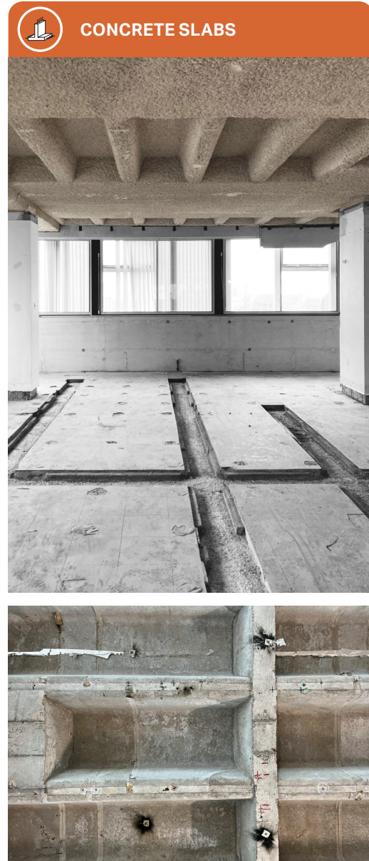
Figure 4.3 Ribbed concrete slabs at Euston Tower
