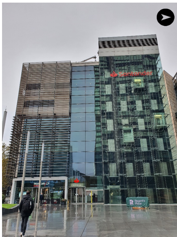
Figure 4: 2 Triton Square looking west from Euston Tower (image taken 10/11/2023, Arup)
