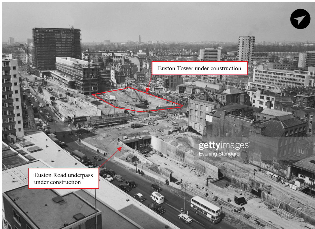
Figure 7 - Euston Road underpass under construction (Evening Standard, 1965)
