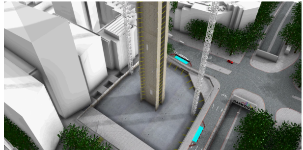
d) completion of floorplate deconstruction to ground level
