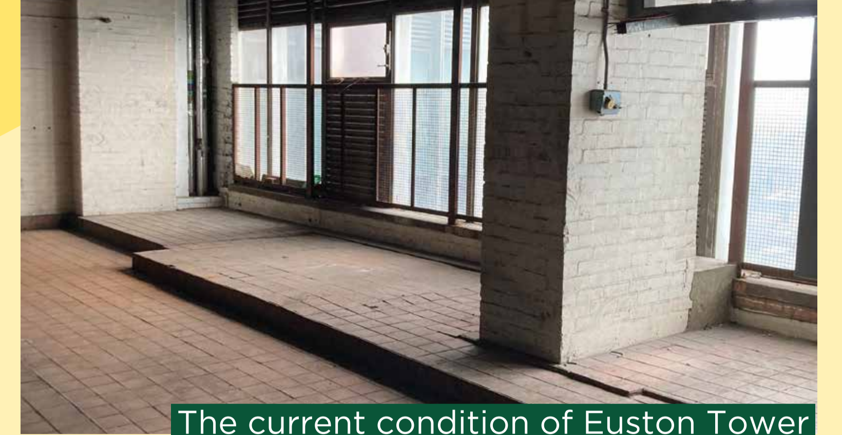
The current condition of Euston Tower
